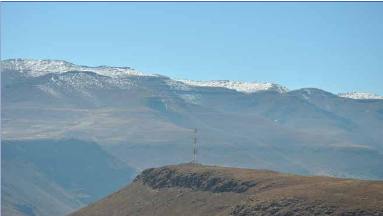
USF funded base transceiver station in Mokhotlong district.
