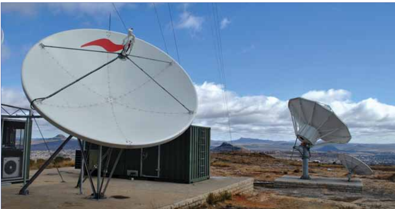
Broadcasting infrastructure of the Lesotho National Broadcasting Service.
