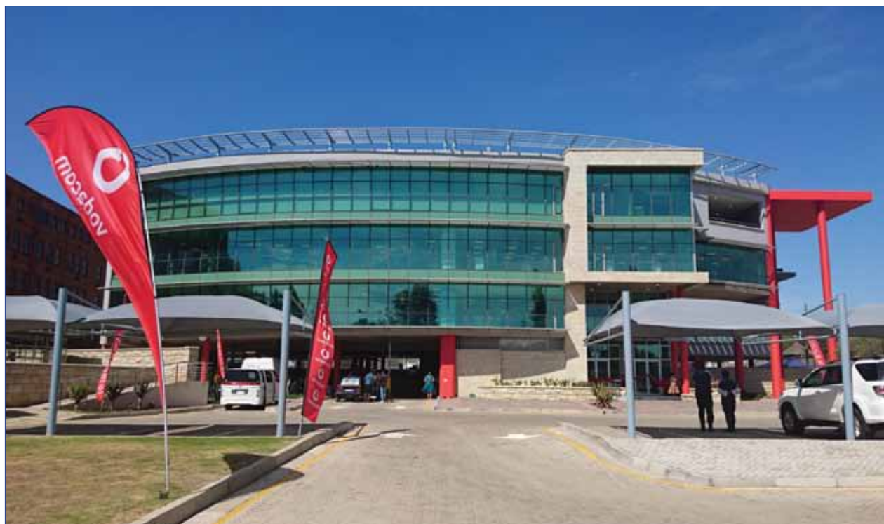
New Vodacom Lesotho head-office in Maseru.
